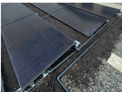
Private pool heating, Switzerland
